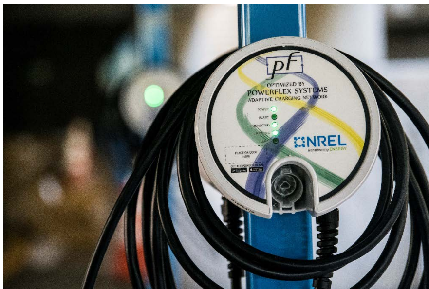
Figure 24. EV chargers on NREL's campus capable of managed charging.
