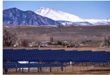
Photo by Werner Slocum, NREL 77079
