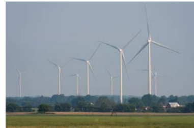
Photo by Werner Slocum, NREL 80135
