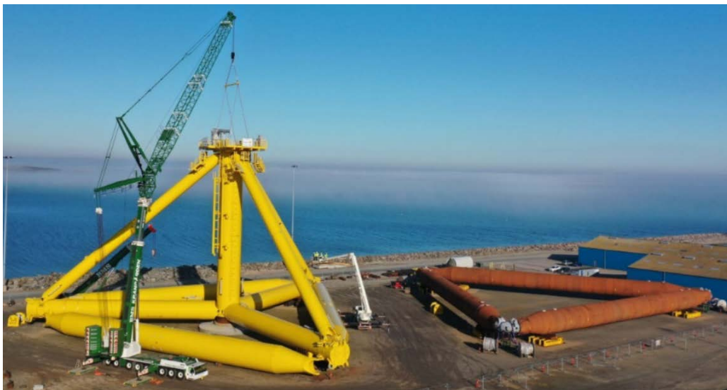
Figure 1. Full-scale TetraSpar assembly in Grenaa, Denmark (Stiesdal Offshore 2023)
