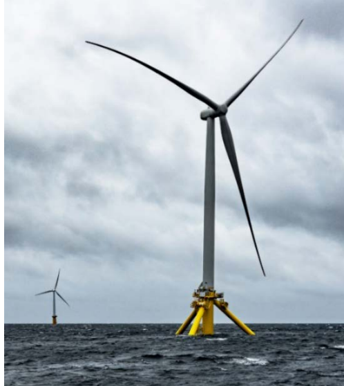
Figure 2. Full-scale TetraSpar operating offshore Karmøy, Norway (Stiesdal Offshore 2023)
