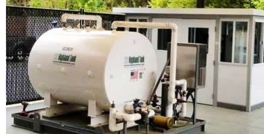
500-gallon heavy fuel oil supply system
