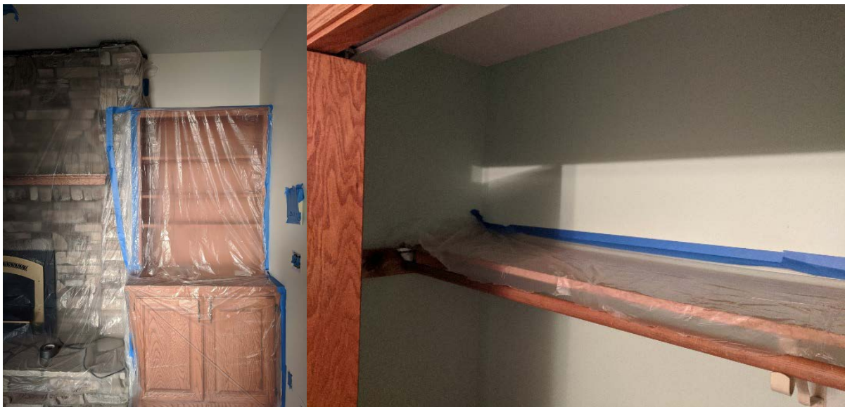
Figure 90. Poly sheet over built-in cabinet and closet shelves
