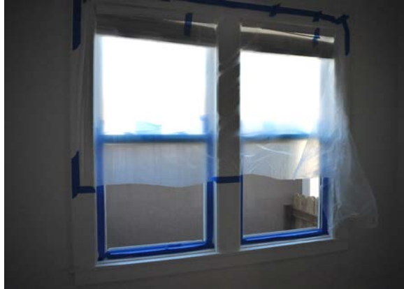
Figure 76. (1) Drape plastic over top half of the window and secure at top
