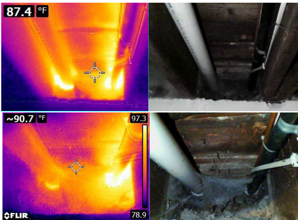
Figure 37. Pre- (top) and post- (bottom) sealing infrared and visual images of basement rim joist showing reduced air leakage through penetrations and joints
