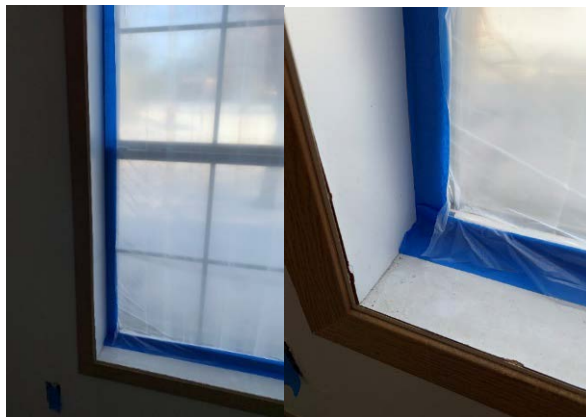
Figure 76. (1) Drape plastic over top half of the window and secure at top
