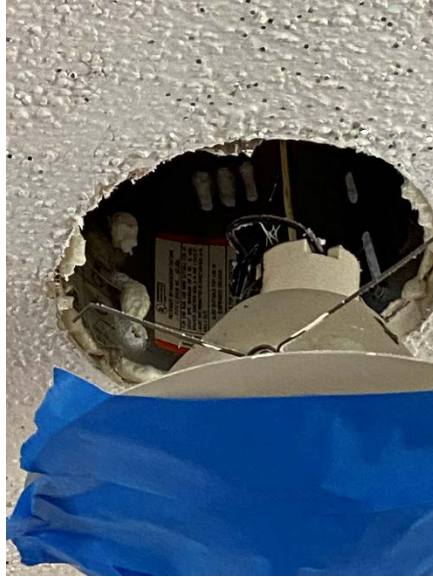
Figure 86. Painter's tape over recessed ceiling fixtures
