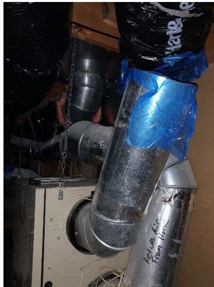
Figure 94. Duct mask to protect HRV disconnected ducts
