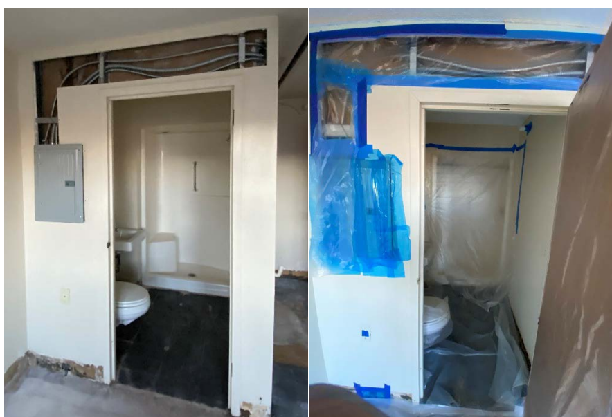
Figure 46. Drywall cut open for renovation (left) and temporary sealing (right)
