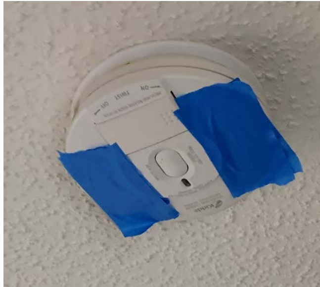
Figure 84. Painter's tape over smoke detector sensors
