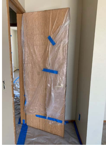
(2) Keep fixture in place. Seal plastic bag to upper edge of fixture.
