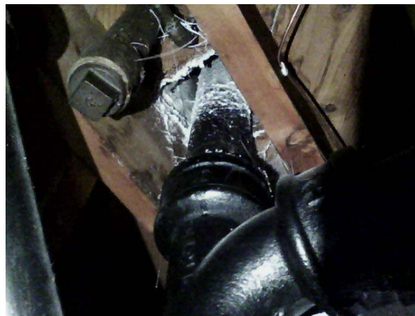
Figure 31. View of plumbing wall from basement where sealant deposition indicates air leakage up the wall
