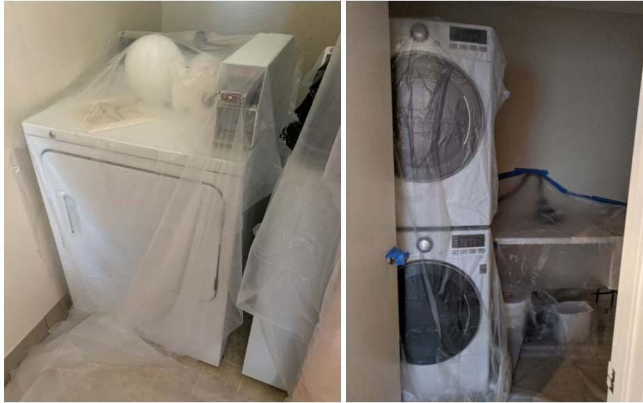
Figure 97. Poly sheet to cover clothes dryer and washer
