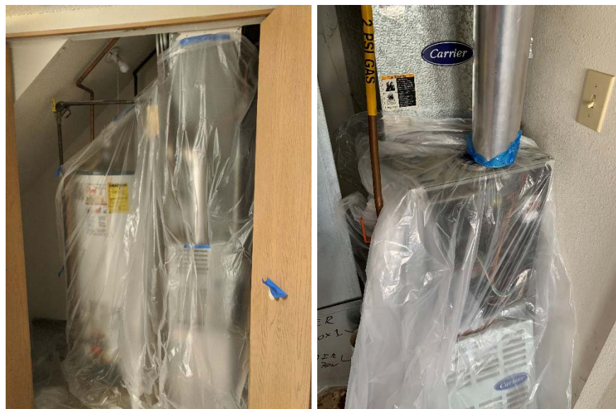
Figure 92. Poly sheet to protect water heater and furnaces
