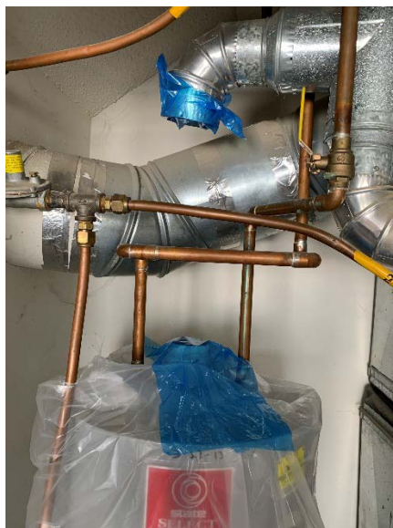
Figure 93. Duct mask and poly sheet to protect water heater vent pipes
