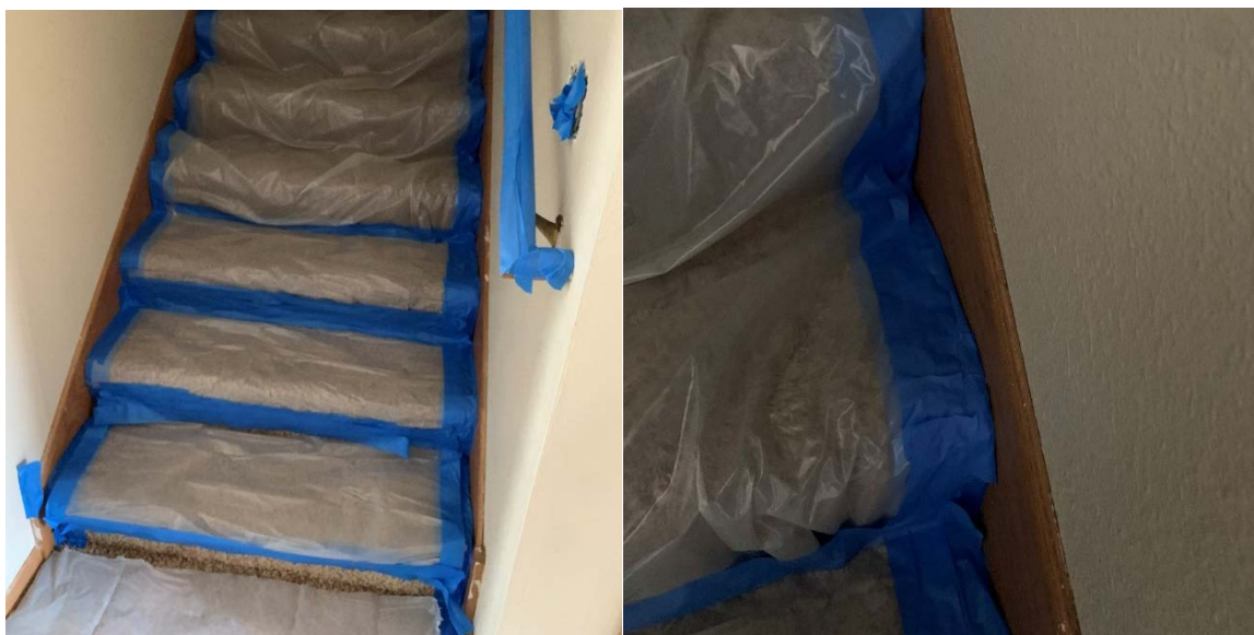
Figure 75. Poly sheet protection for flooring over slab or above finished space
