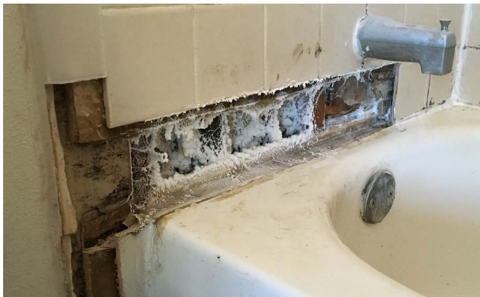
Figure 20. Construction in bathroom exposing the wall cavity where significant sealant collected due to high amounts of leakage
