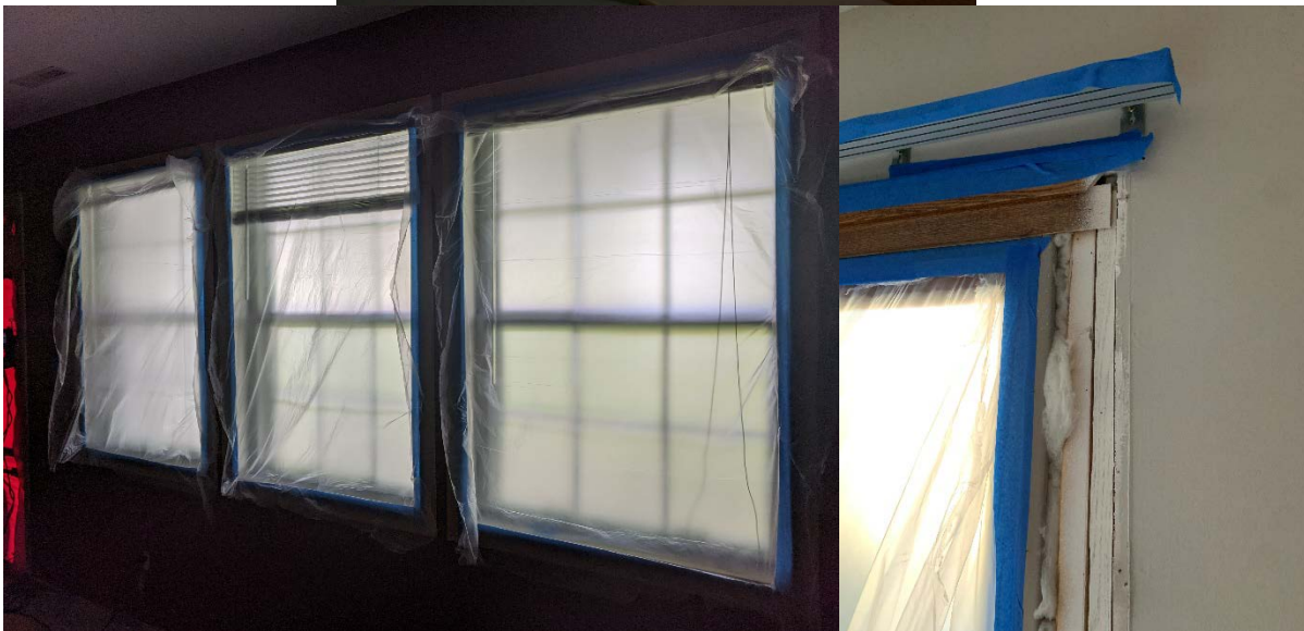
Figure 77. (2) Cover entire pane with plastic. Tape at sides and top, but leave open at bottom. Permanent window fixtures (e.g., blinds, curtains) need to be protected by plastic and painter's tape
