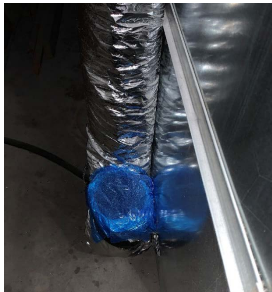
Figure 95. Duct mask to protect combustion air duct opening
