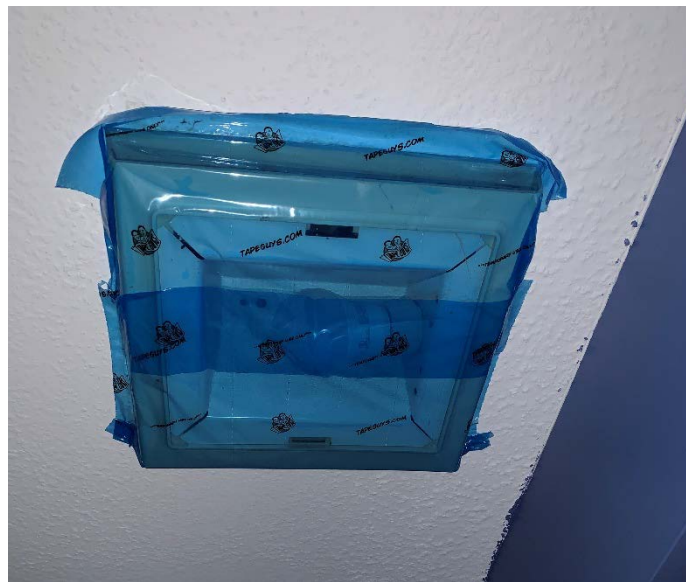
Figure 96. Duct mask to protect ceiling exhaust fan grille
