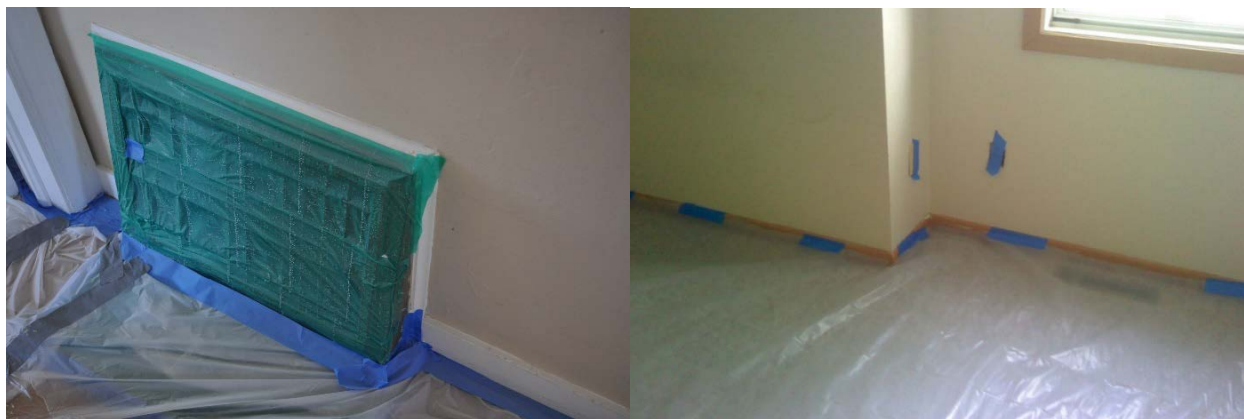
Figure 91. Poly sheet and duct mask over air distribution system grilles
