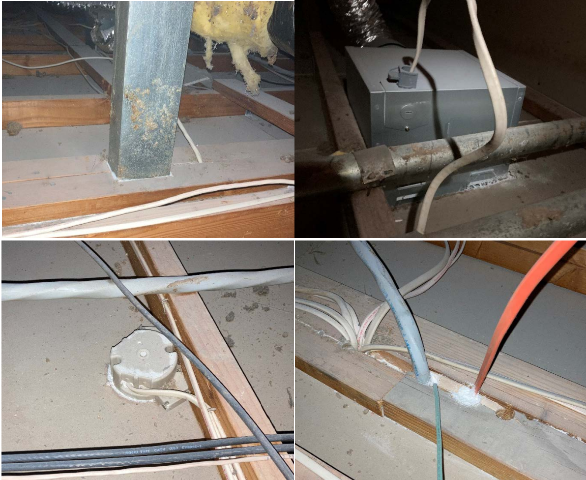
Figure 55. Attic seals made at duct (upper left), fan housing (upper right), ceiling light box (lower left), and wire penetrations (lower right)
