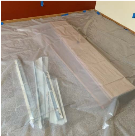
(1) Remove fixture from ceiling and place bag over fixture.
