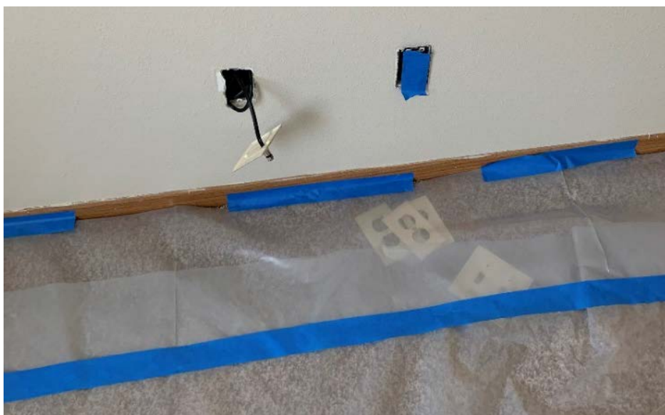
Figure 73. Poly sheet protection for flooring over slab or above finished space
