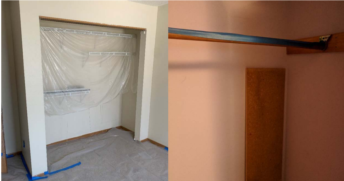
Figure 89. Poly sheet and painter's tape over closet hardware
