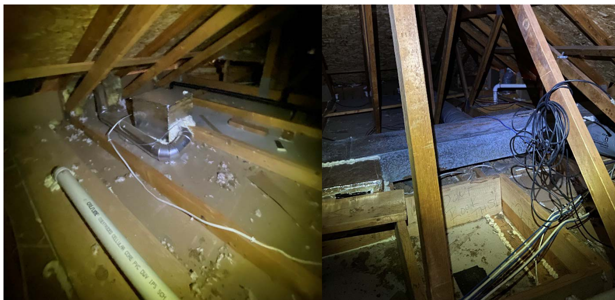
Figure 58. Manual sealing performed before aerosol sealing
