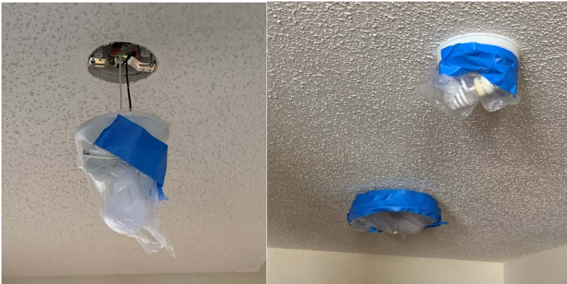
Figure 85. (Left) Remove fixture from ceiling and place bag over fixture. (Right) Keep fixture in place. Seal plastic bag to upper edge of fixture
