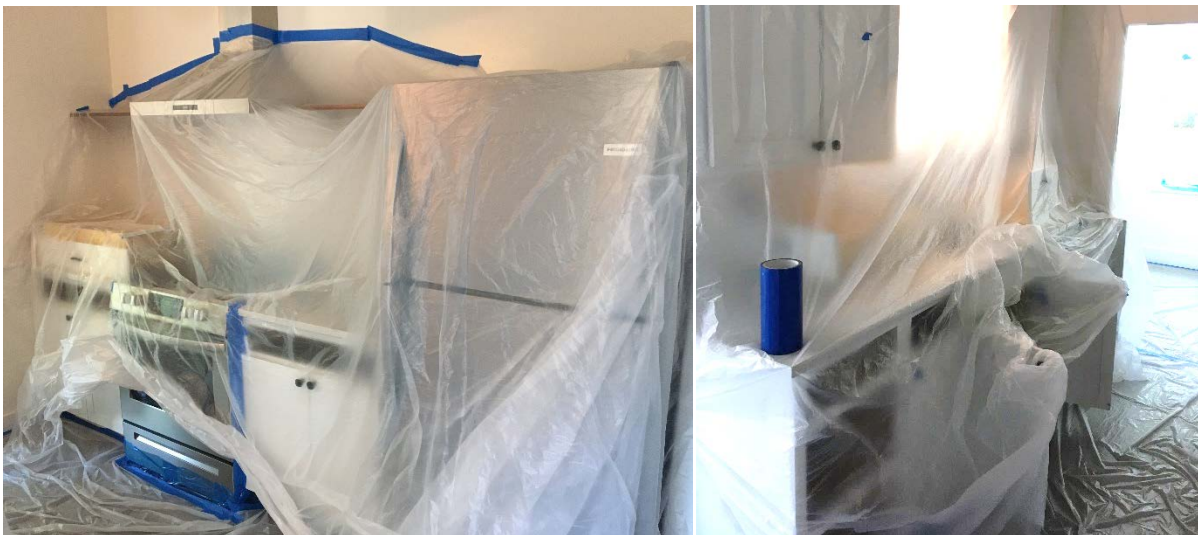
Figure 3. Kitchen appliances and cabinets are covered for sealing. The photo on right shows cabinets opened to allow aerosol to seal plumbing penetrations and outlets below the sink
