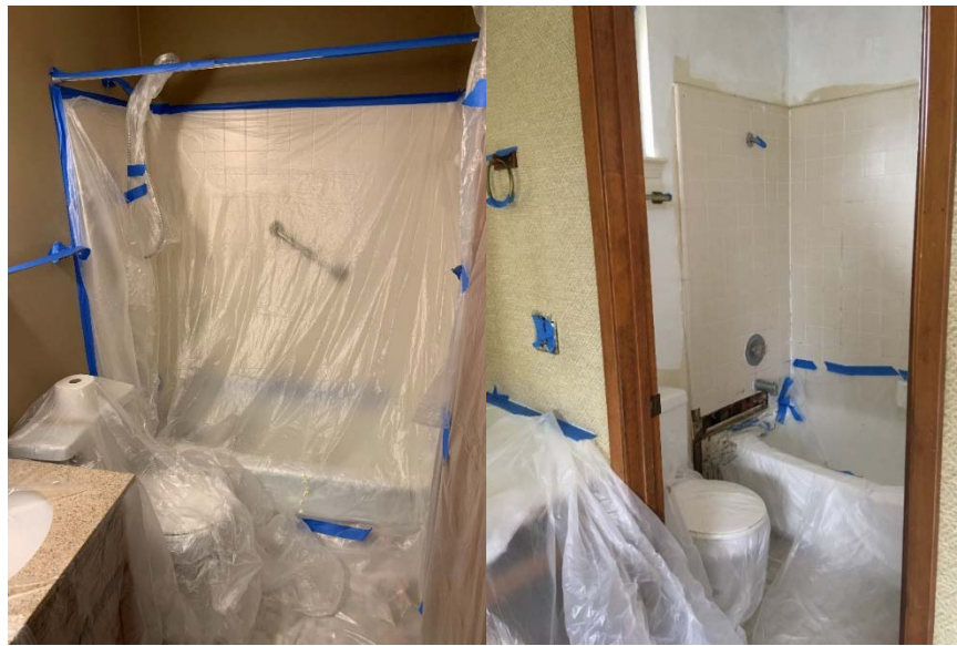
Figure 80. (Left) Cover walls with plastic. Drape over tub so that upper edge of tub is covered. Leave open at bottom. (Right) Tape plastic sheet to wall surrounding the tub about a foot above the tub and drape the plastic over the tub so that the upper edge is covered. Leave open at bottom
