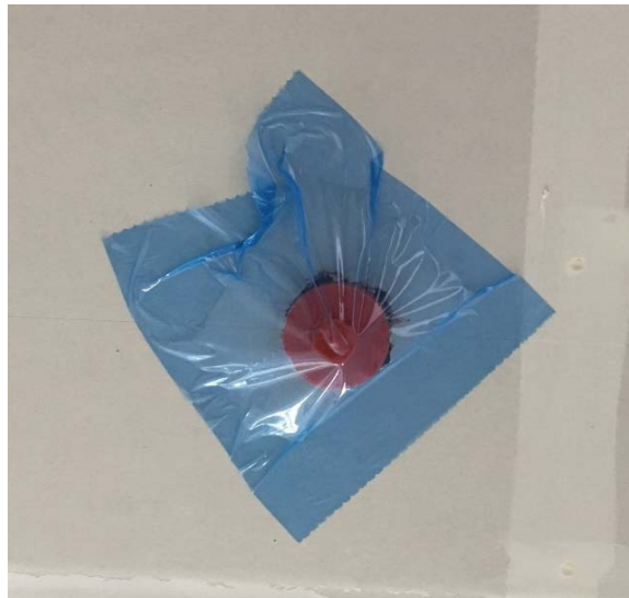
Figure 82. Protect sprinkler heads from sealant intrusion
