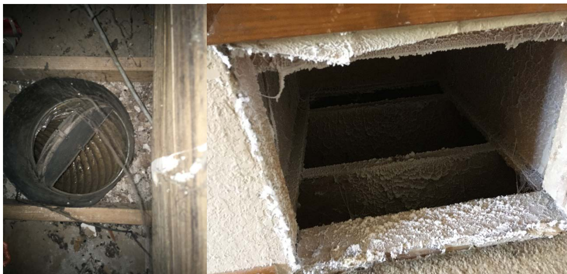
Figure 19. Return plenum opening inside wall cavity (left) and return entrance showing significant deposition (right)
