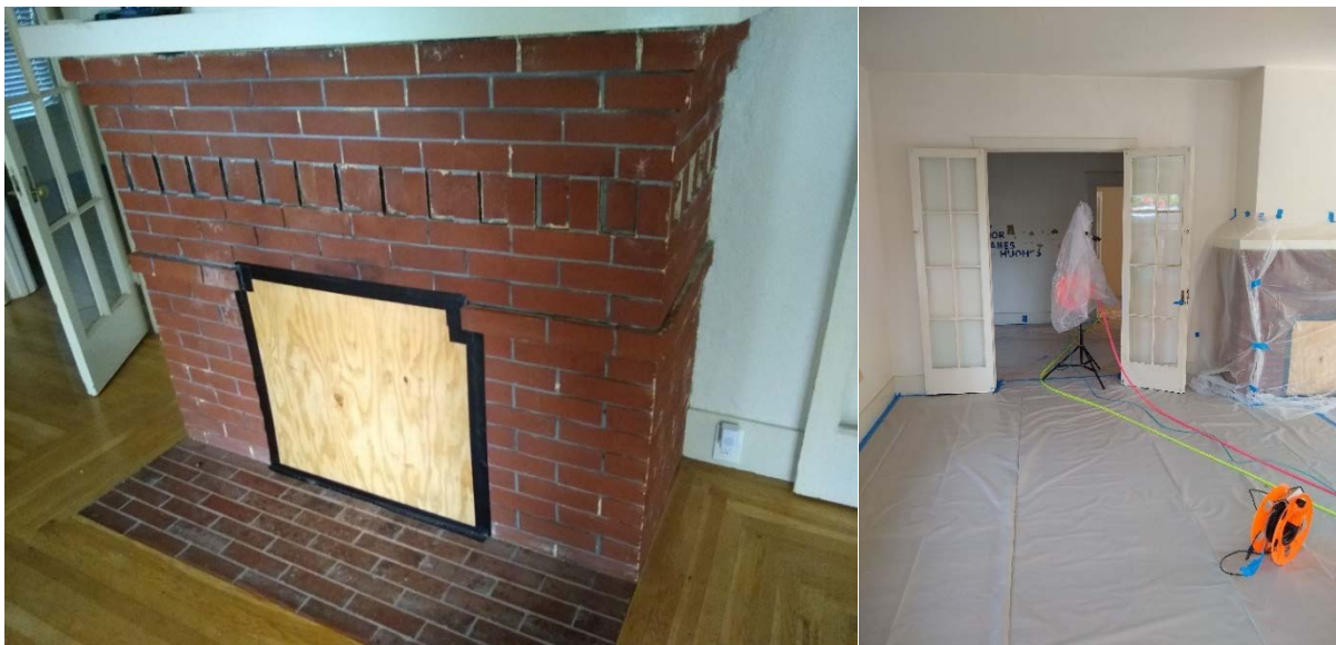
Figure 98. Plywood and poly sheet to protect fireplace opening
