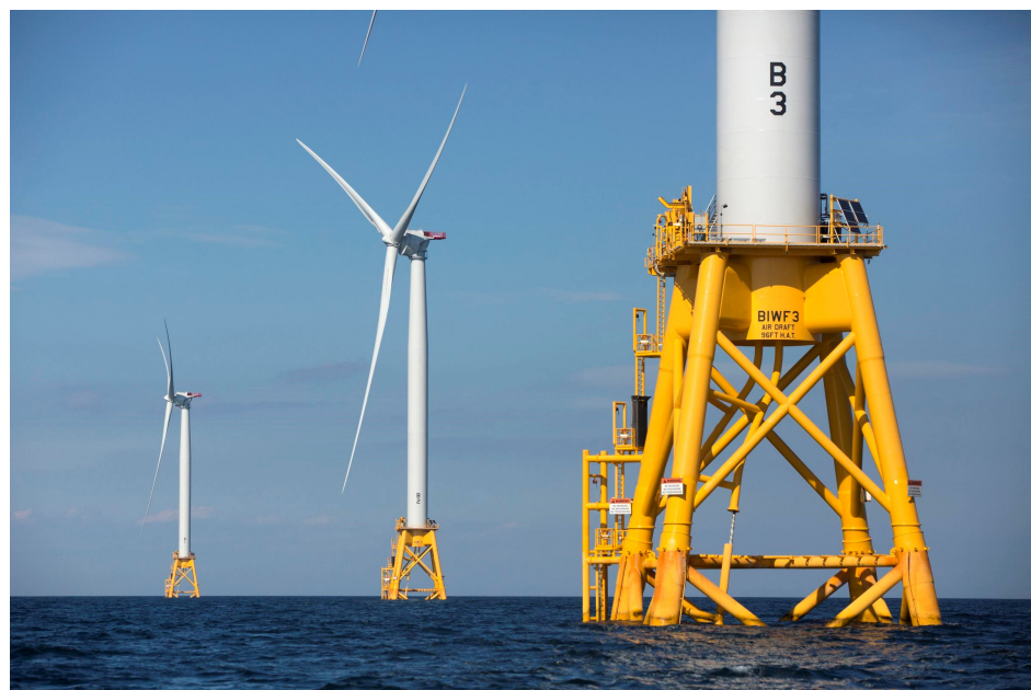
Figure 2. Wind turbines B1–B3 (from left to right) standing in the Block Island Wind Farm, RI, USA (Photo: Michael Dwyer).
