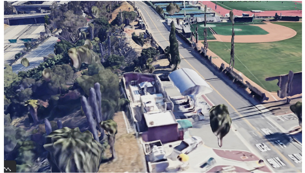
Aerial view of fueling station. Picture from Google Streetview
