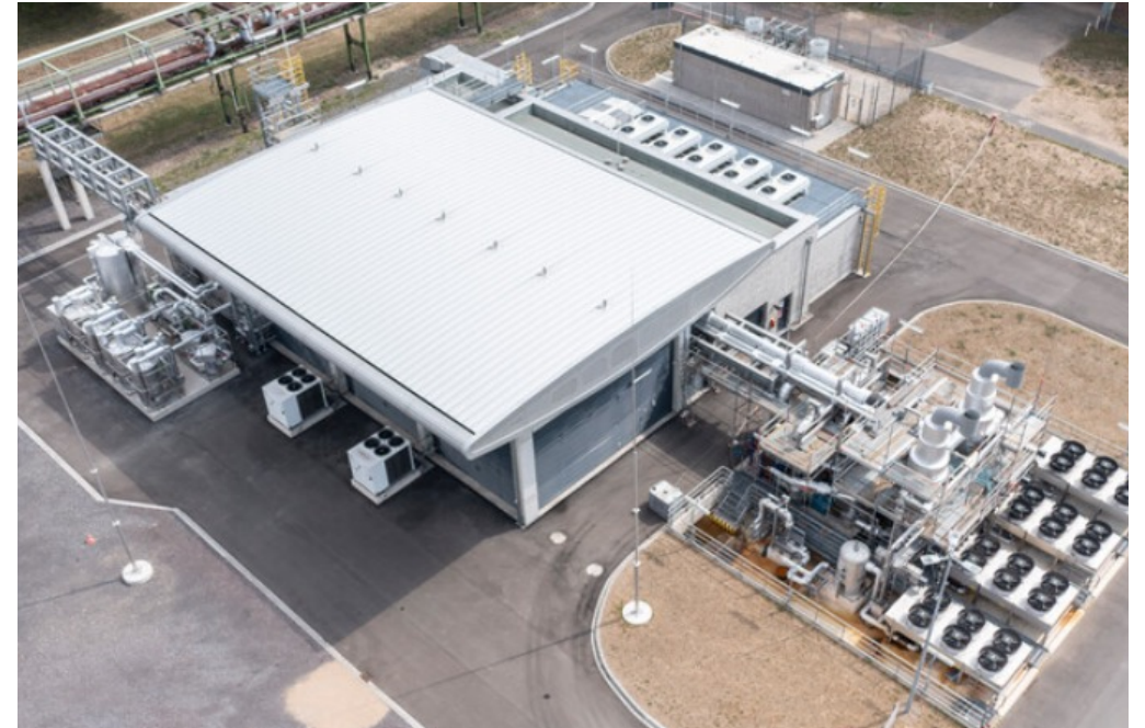
Birds eye view of Shell's PEM green hydrogen production facility. Image by Shell Photographic Services.
