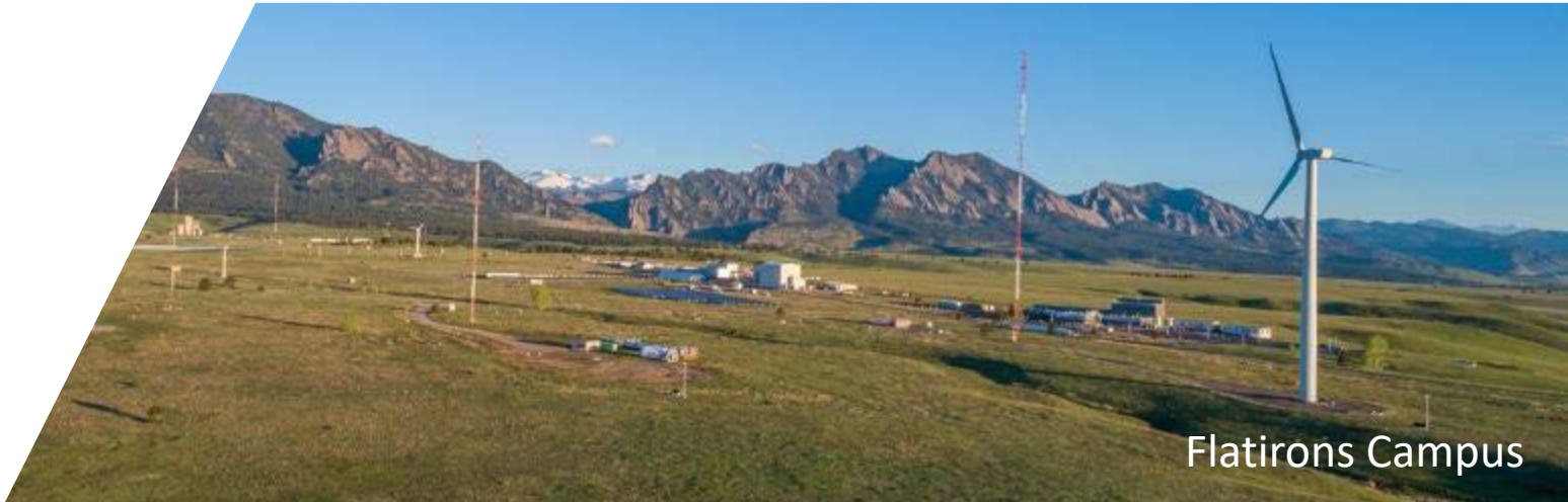
Energy Systems Integration Facility
