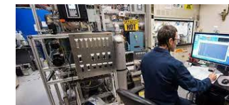
2" Fluidized Bed Reactor (2FBR)
