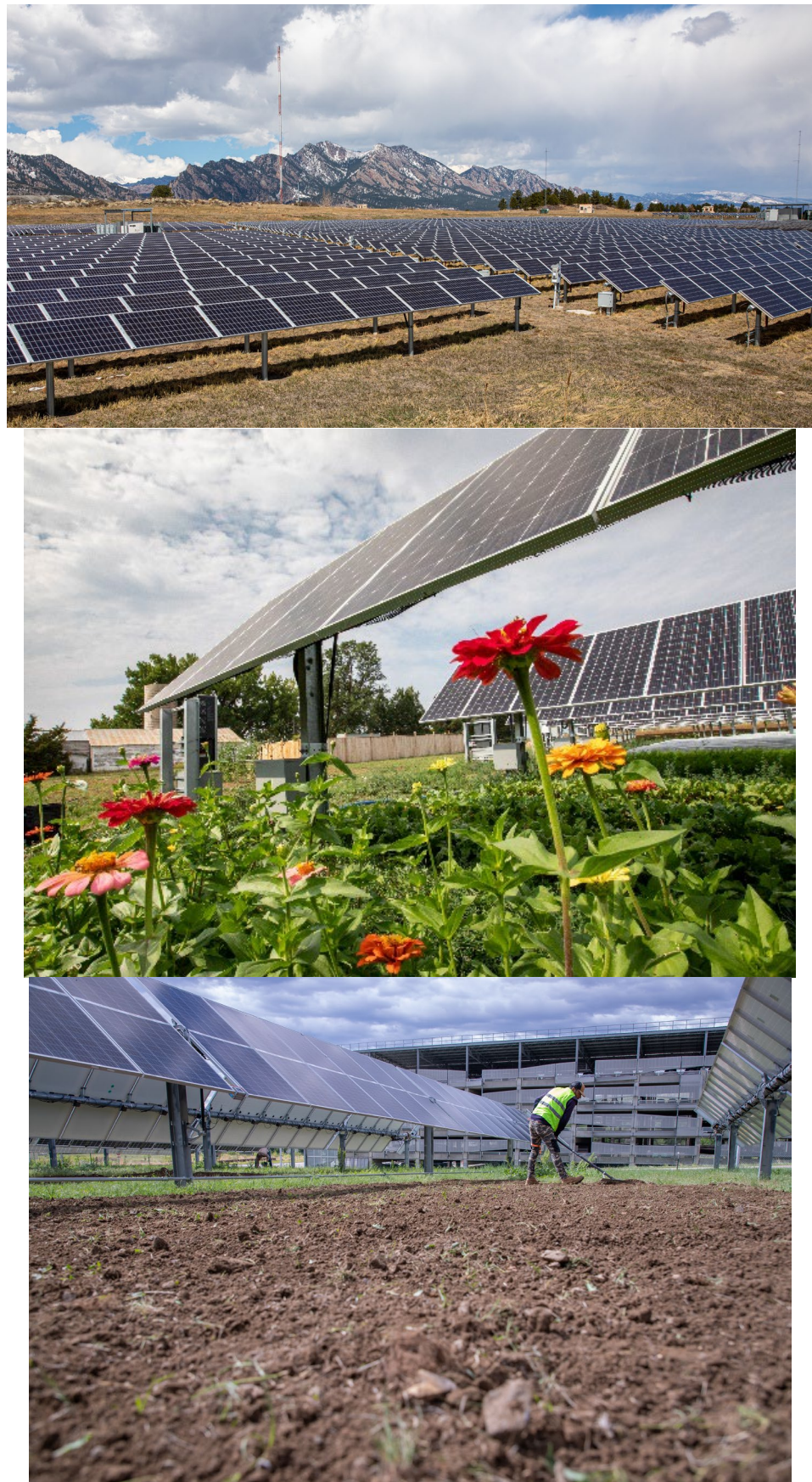
Figure 2. Turf grass ( top ), pollinator habitat ( middle ), and bare ground ( bottom ) under solar PV systems. ( top ) Photo by Werner Slocum, NREL 65337, ( middle ) photo by Werner Slocum, NREL 65625, and ( bottom ) photo by Joe DelNero, NREL 68429 [23].
