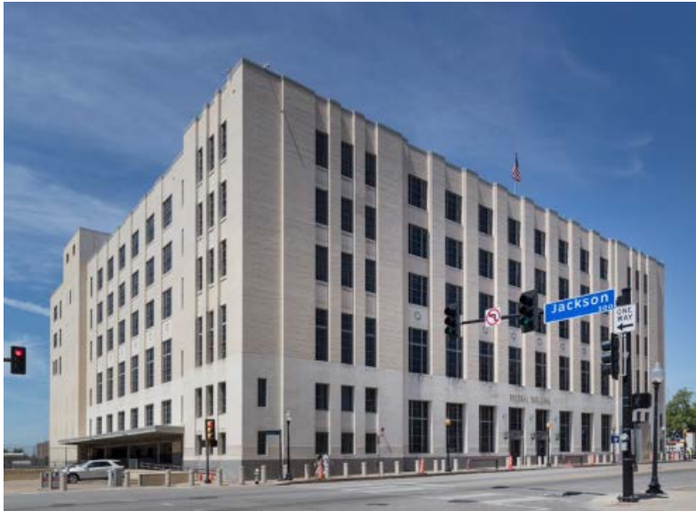
Figure 2: Terminal Annex Federal Building
