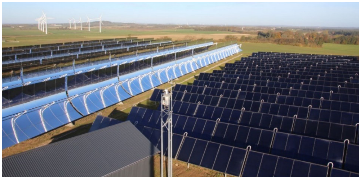
Figure 5. Tårs, Denmark hybrid RTES site utilizing parabolic trough and flat plate collectors for district heat provision (Aalborg CSP 2015b).
