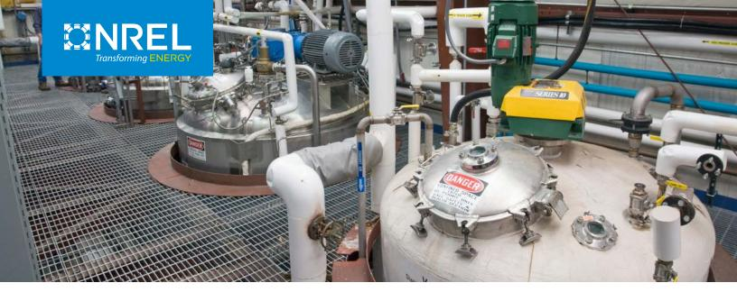
NREL's DMR process reinvents biomass pretreatment to yield larger quantities of cheap lignocellulosic sugars—choice ingredients for making low-carbon fuels, chemicals, and materials. *Photo from NREL, 16332*
