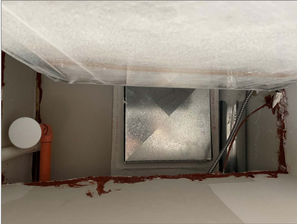
Figure 9. Unsealed penetration into above-ceiling supply and exhaust duct chase
