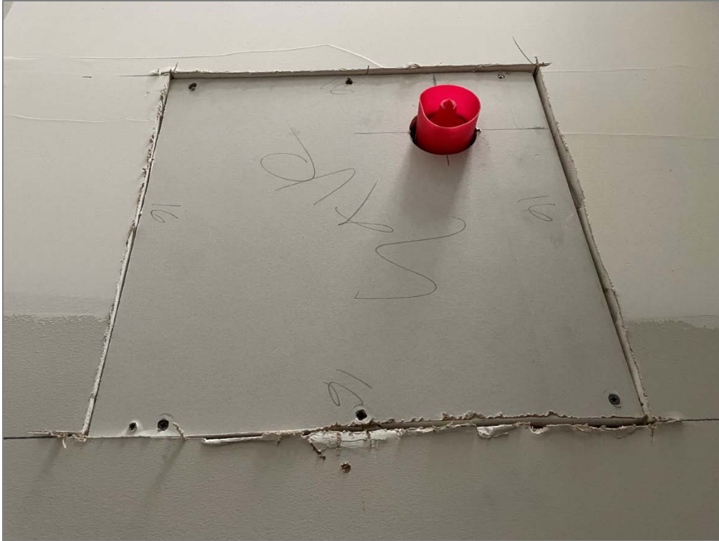
Figure 7. Unsealed ceiling access
