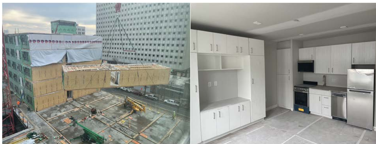
Figure 1. Prefabricated multifamily building modules
