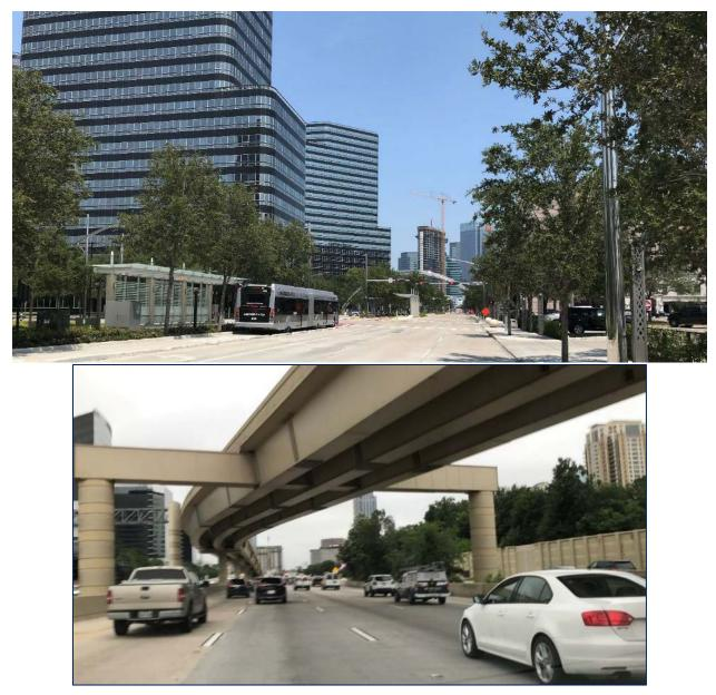
Figure 4-5. The Silver Line BRT alignment transitions from aerial on the north end to at-grade on the south end through the Uptown district. Top: At-grade segment of the BRT Sliver Line alignment passes through office and residential towers that span 50 years of development activity. Bottom: View looking south along the IH-610 West Loop freeway, where aerial BRT alignment transitions to the center of the freeway to descend to grade.
