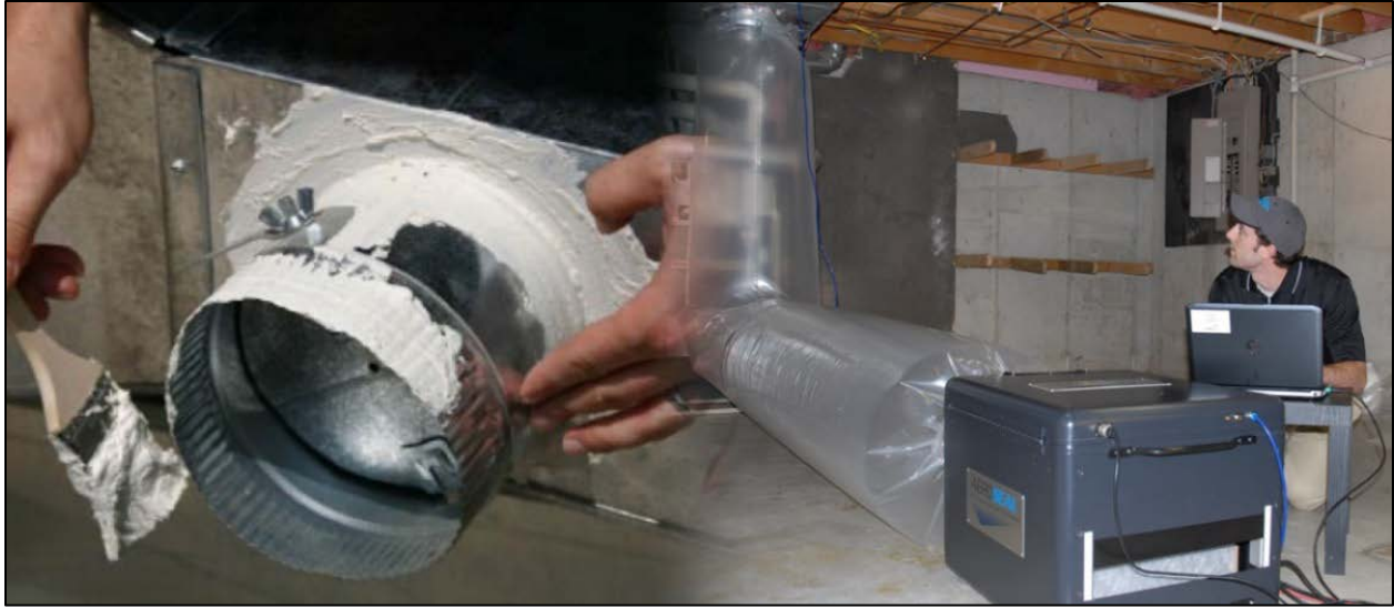
Figure 1. Photos of manual sealing (left) and aerosol-based sealing (right)
