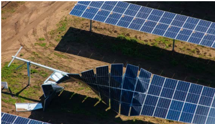
Wind Damage – Long read: What broke at Oakey – pv magazine Australia (pv-magazine-australia.com)
