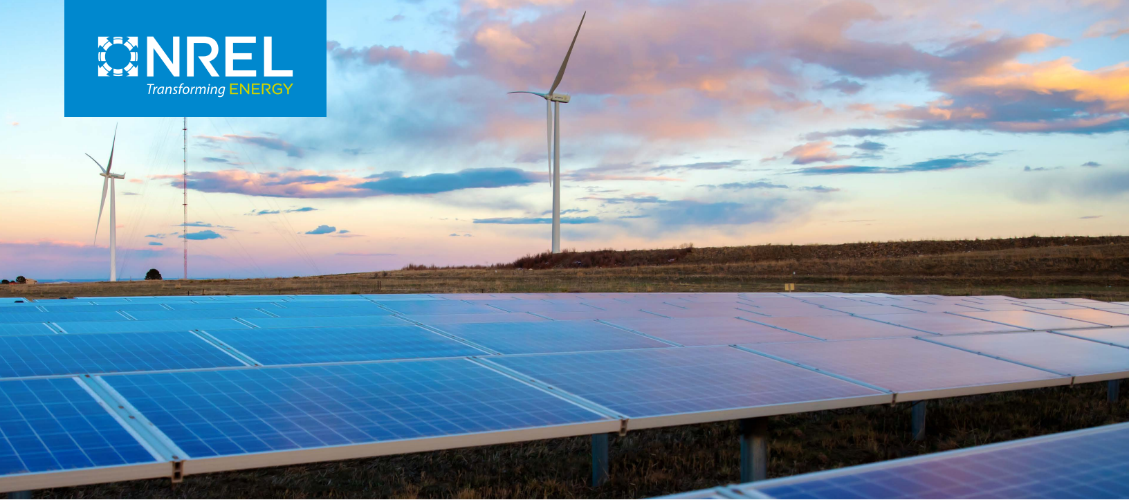
Photo by Werner Slocum, NREL 65320
