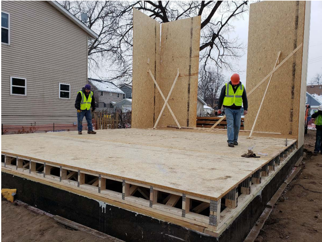
Figure B-5. Exterior vertical panels are set (plumb, square, and level) at corners
