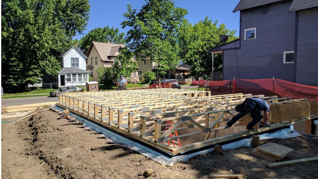
Figure B-3. Receiver plate and first floor joists installed
