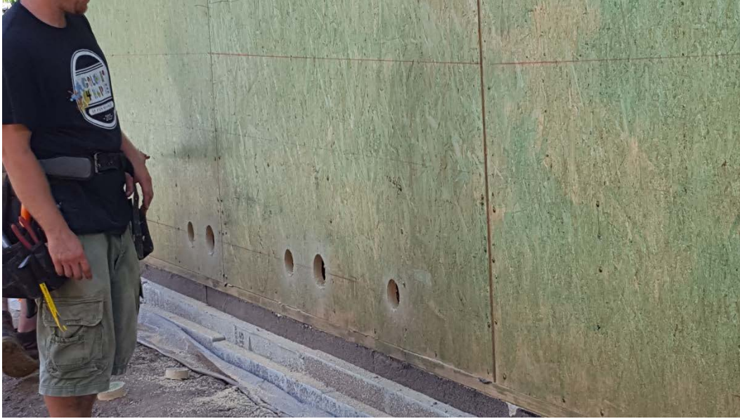
Figure B-13. All penetrations (with a couple of spares) are pre-located and cut
