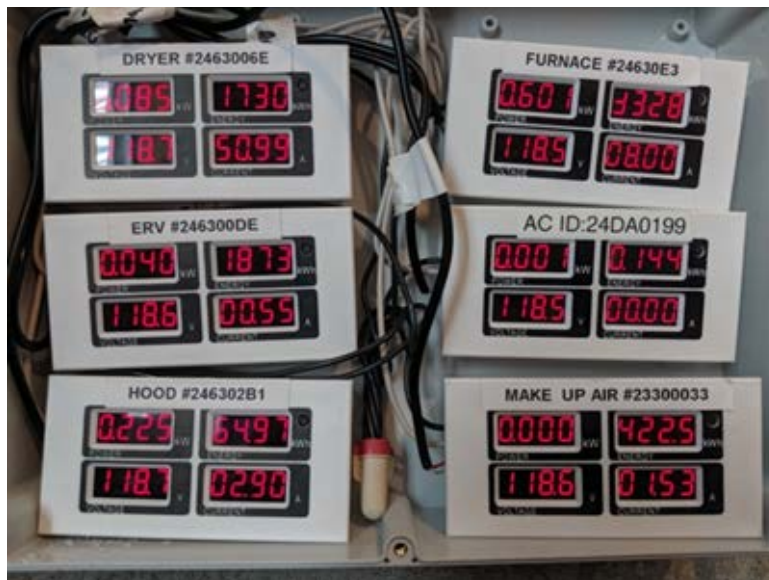
Figure 6. Electric current monitors
