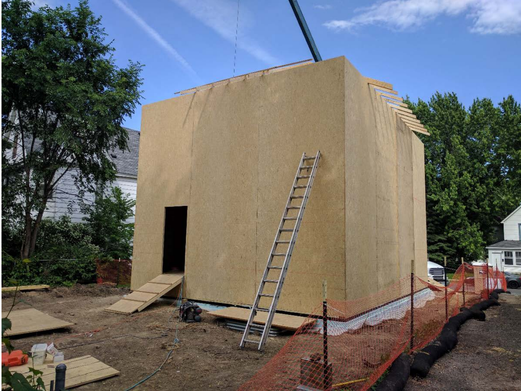
Figure B-9. Completed exterior vertical wall panels (with cut rear entry)
