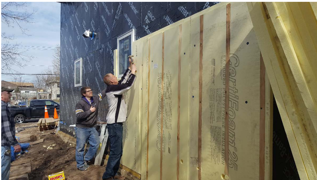
Figure B-16. Installing exterior control layers with embedded furring strip for vinyl cladding
