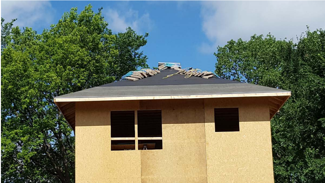
Figure B-11. Installation of roof sheathing, building paper, and shingles (dried-in)
