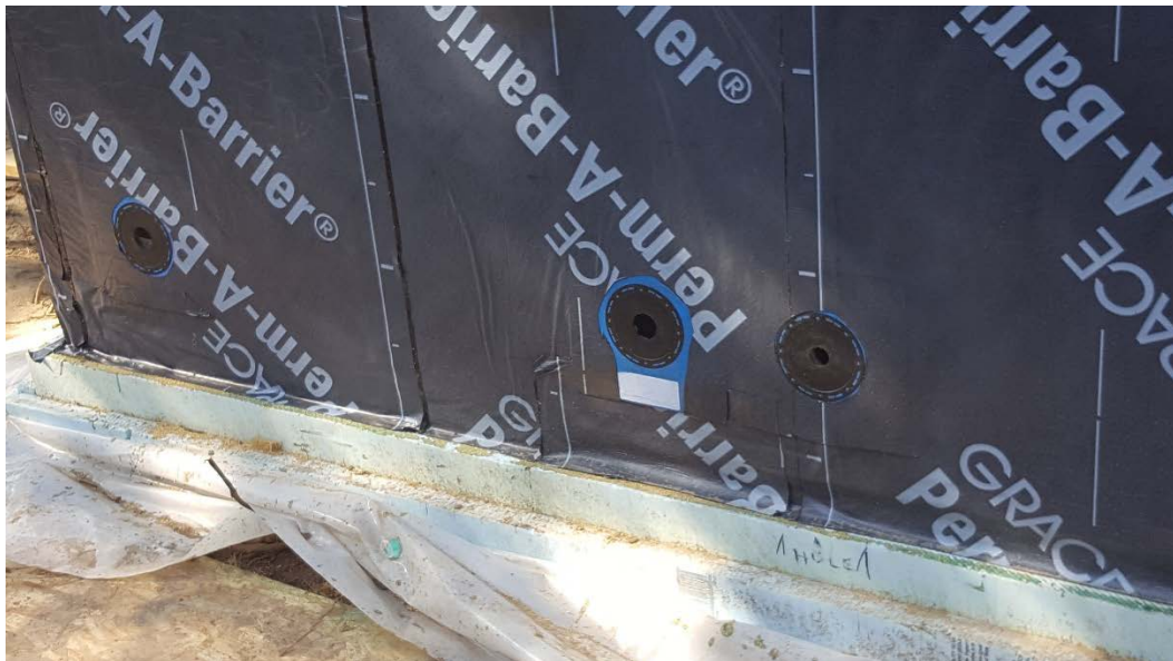
Figure B-14. All penetrations are integrated with the air, water, and vapor control membrane
