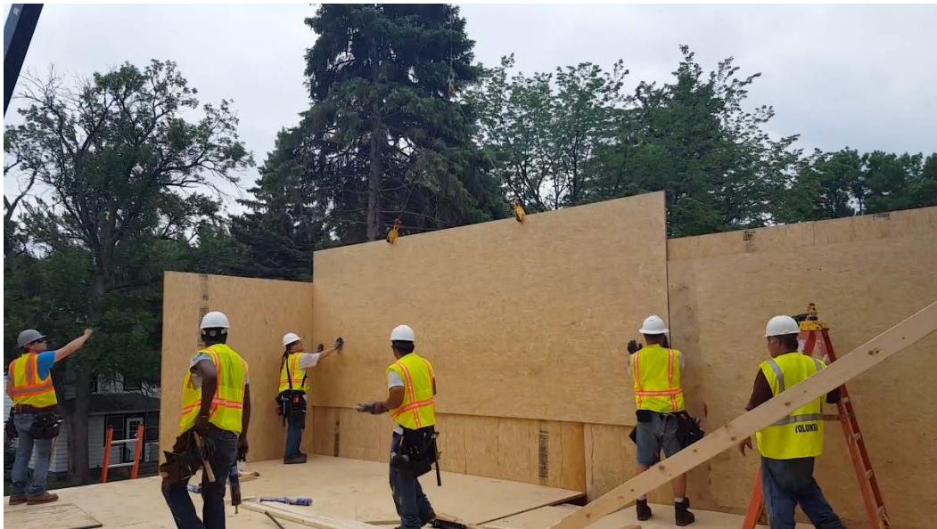
Figure B-8. Installation of second floor interior horizontal panels
