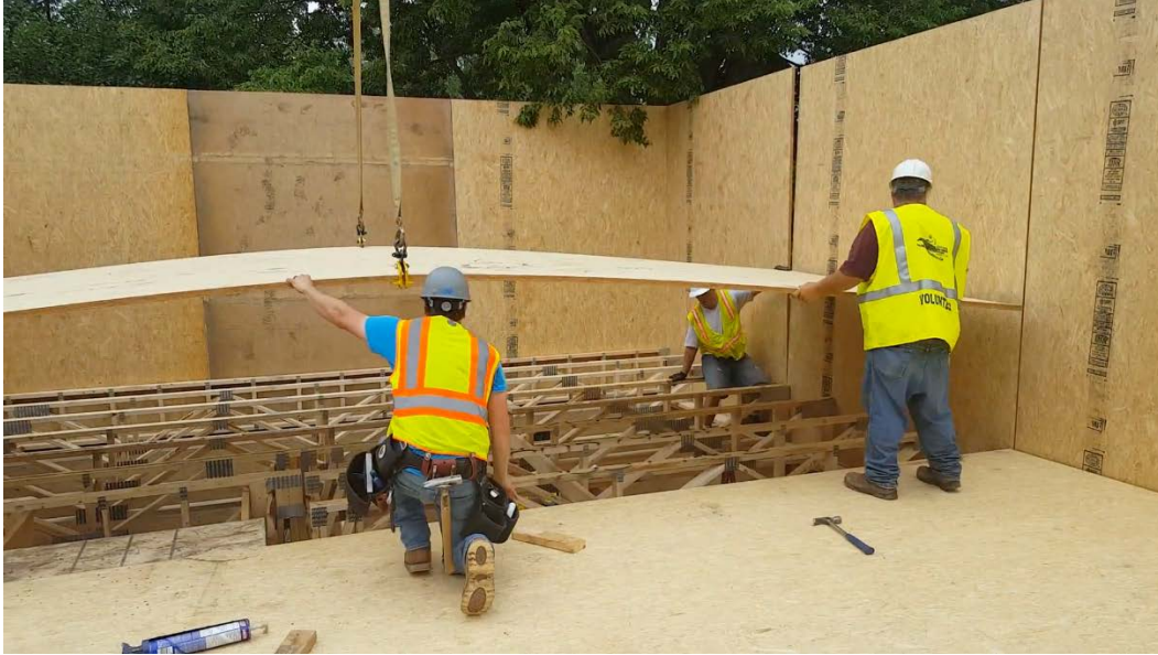
Figure B-7. Installation of second floor joists and sheathing
