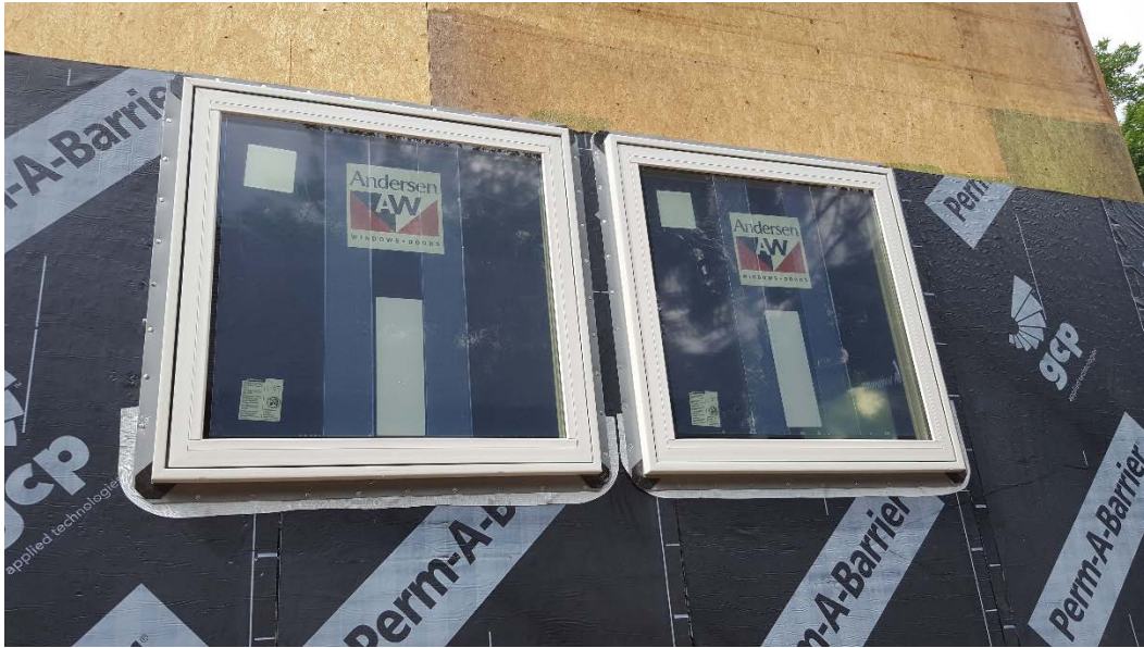
Figure B-15. Lower-level window installation integrated with air, water, and vapor control membrane
