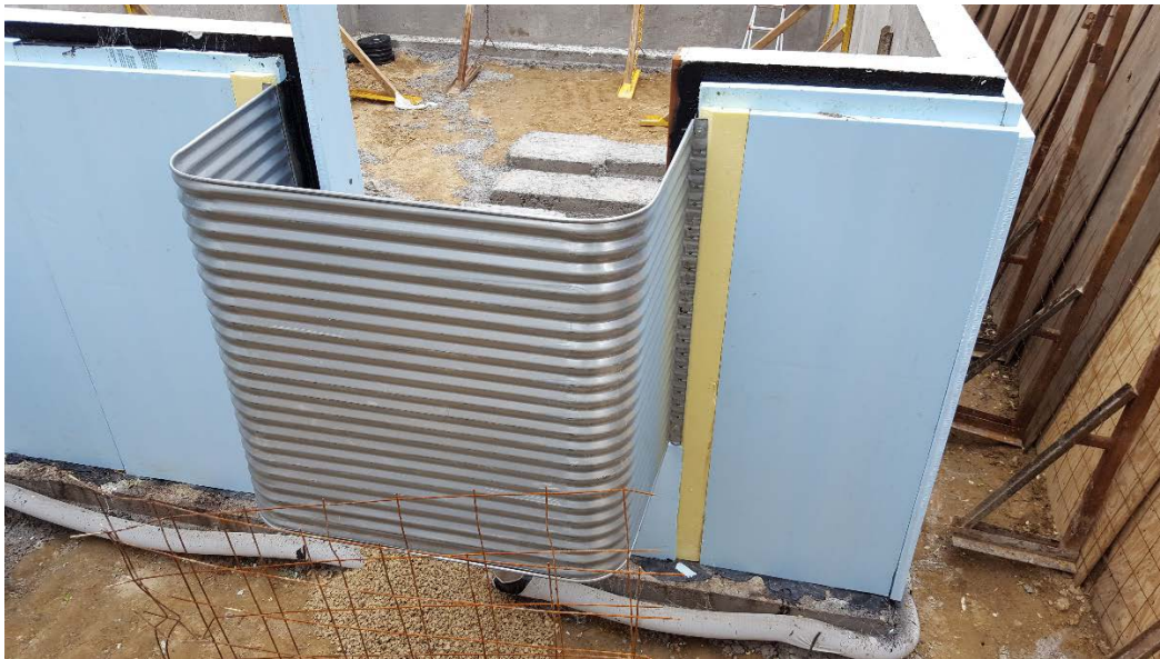
Figure B-2. Window well for basement egress integrated with control layers
