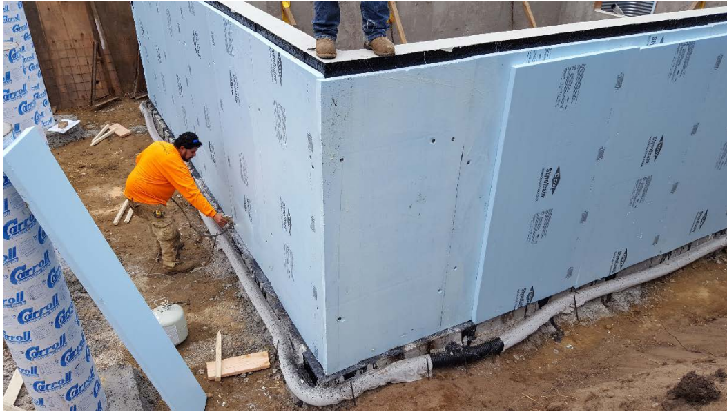
Figure B-1. Basement foundation with control layers
