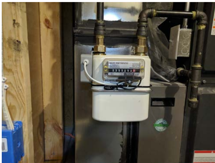
Figure 7. Typical natural gas submeter installation
