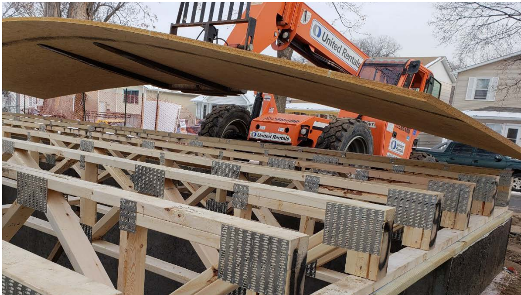
Figure B-4. First floor sheathing installation
