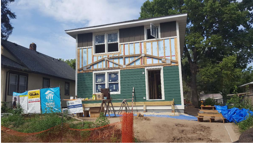
Figure B-17. Furring strips over foam for fiber-cement cladding installation (note porch connection)
