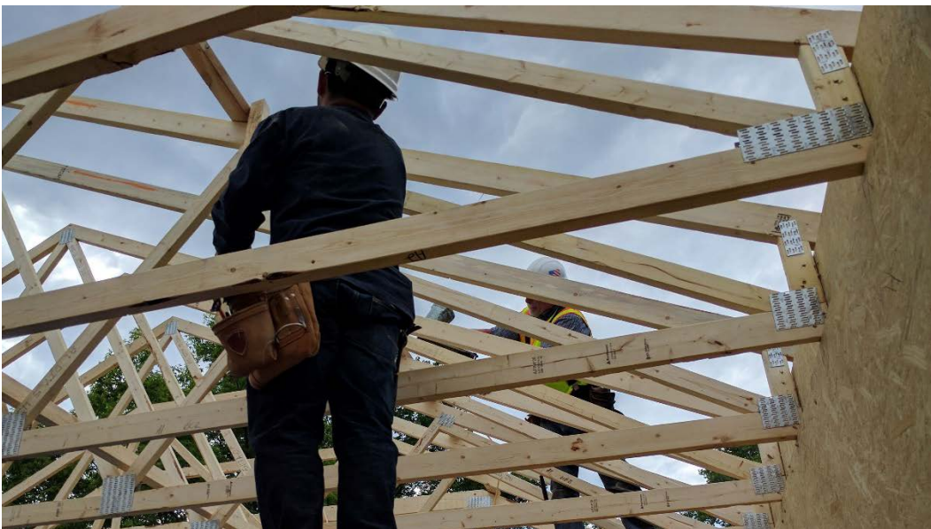
Figure B-10. Roof trusses are set inside the vertical panels and on the horizontal panels
