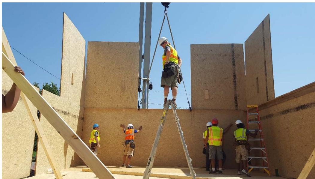
Figure B-6. Installing first floor interior horizontal panels
