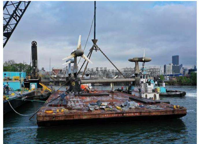
In May 2021, Verdant Power performed a retrieve-and-replace operation, during which one of the turbine rotors was replaced with a rotor comprising three thermoplastic blades manufactured by NREL. *Photo from Paul Komosinski, Verdant Power.*
