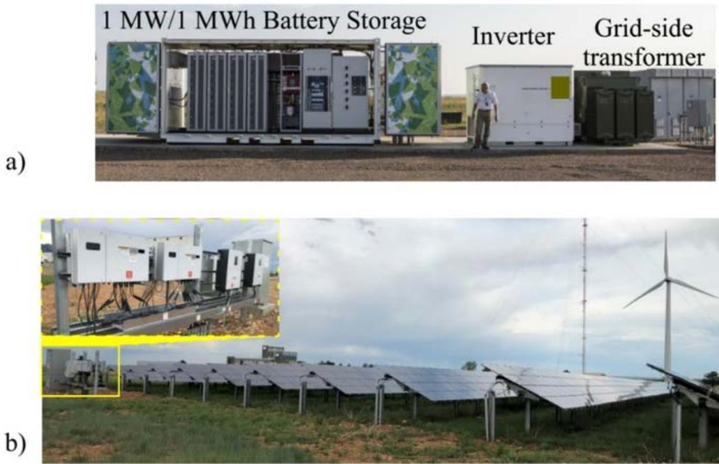
Figure 77. Inverters for impedance characterization: the (a) 2.2-MVA inverter interfacing the 1-MW/1-MWh BESS and the (b) 430-kW PV plant with six string inverters. *Photos by NREL*
