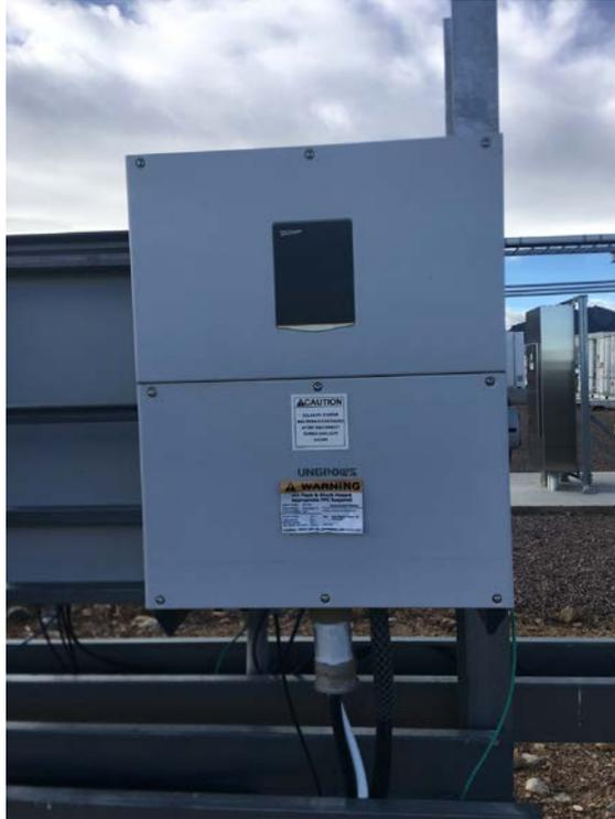
**Figure 13. A 125-kVA string inverter (Sungrow SG125HV)**
