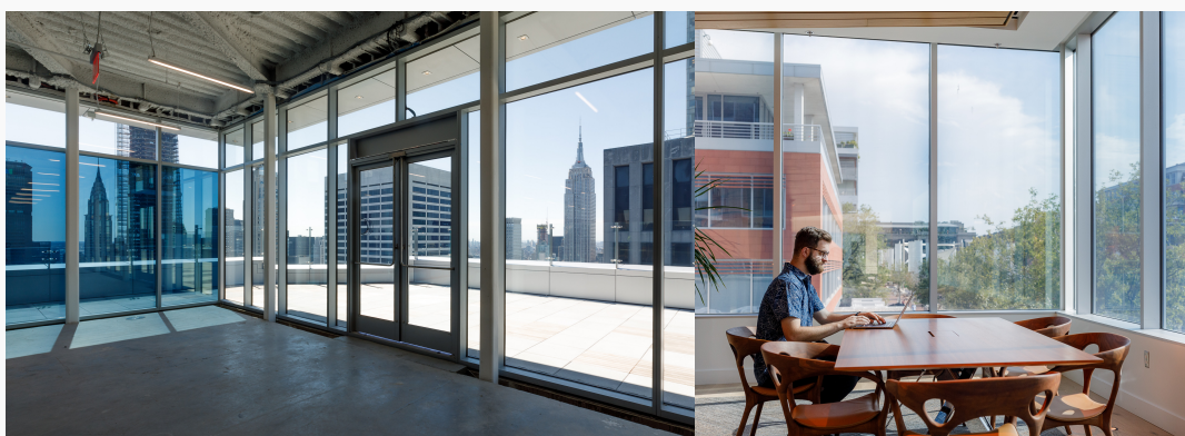
Figure 10. Dynamic glazing can be adjusted to a range of levels to manage occupant thermal and optical comfort while maintaining views to the outdoors.
