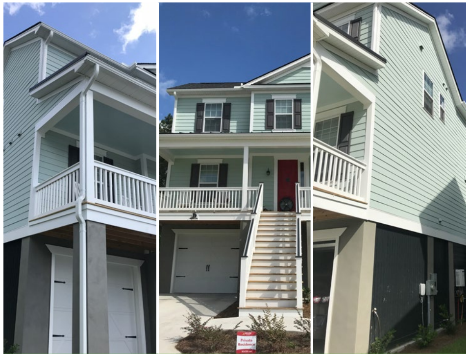
Figure 1. New construction test homes each featured a two-story elevated plan built on approximately 9-ft concrete piers, as they are located in a flood zone. Homes were selected for their similar layout and square footage (2,300 ± 100 ft 2 ).
