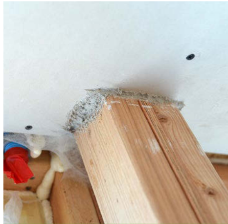
Aerosol sealing installation on a single-family home including examples of seals formed. Photos from UC Davis WCEC
