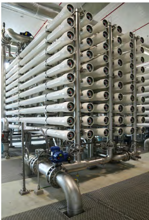
Figure 4. Reverse osmosis systems used at the KBH Desalination Plant in El Paso, Texas 30
