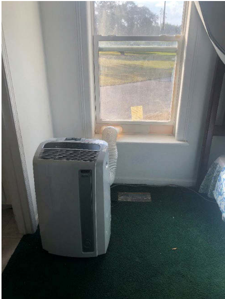
Figure 3. A portable air conditioner can be used to aid with containment, and provide comfort to the isolation zone, because it is recommended that supply and return grilles in the isolation zone be closed off during containment. Photo courtesy of FSEC
