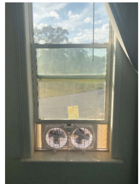
Figure 2. An inexpensive window fan can aid with containment.
