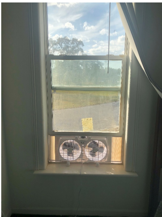
Figure A1. Window fan installed in the IZ exhausting air to outdoors
