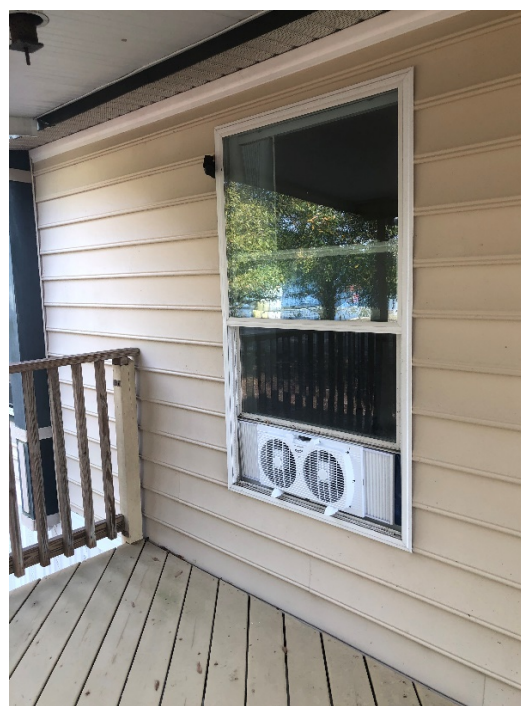
Figure A2. Window fan installed in MZ providing outdoor air into home
