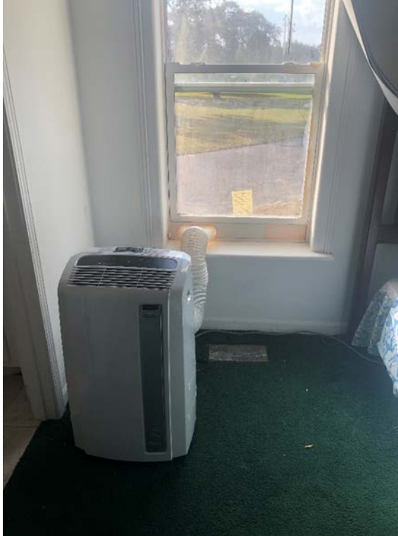
Figure A3. Portable air conditioner in IZ with unit exhaust through window
