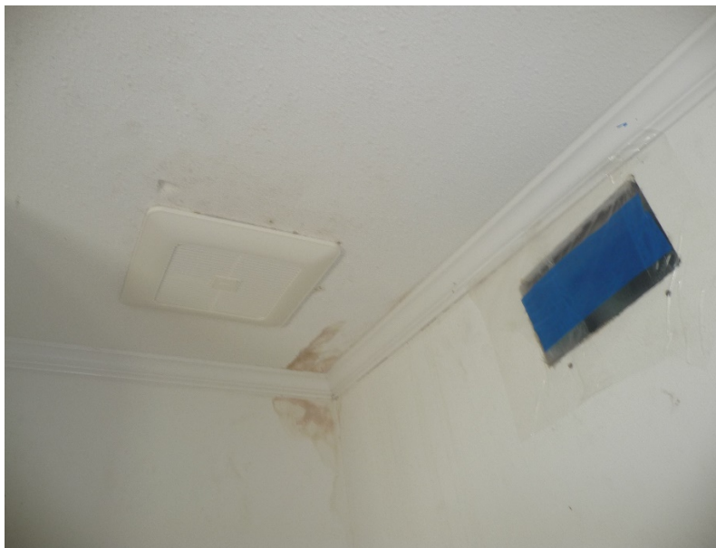
Figure A5. Bathroom exhaust fan in IZ shown next to a sealed off supply grille
