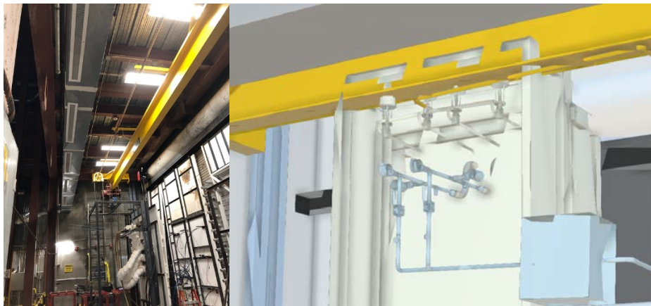
Figure 60. Interference of sodium receiver housing and existing crane, which will be removed during initial site construction. (Left) site photo; (Right) 3D render of proposed sodium-receiver housing overlaying with the crane
