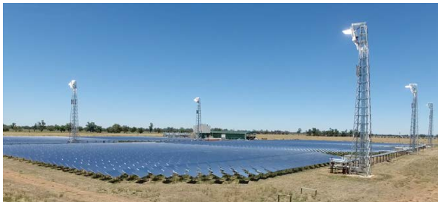
Figure 64. Vast Solar's 5-MW Jemalong pilot plant has derisked sodium handling in preparation for their proposed Mt. Isa project
