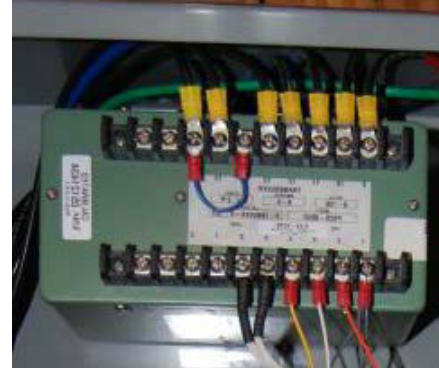
Power, VA, volts transducer (external CTs)
