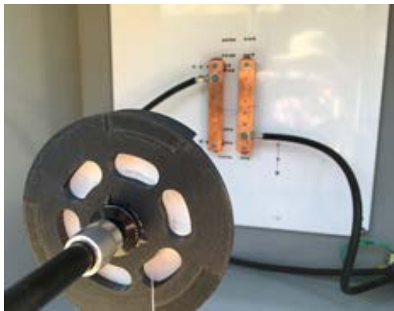
Fig. 8 - Vertical Flat Bus Configuration as tested (NREL)
