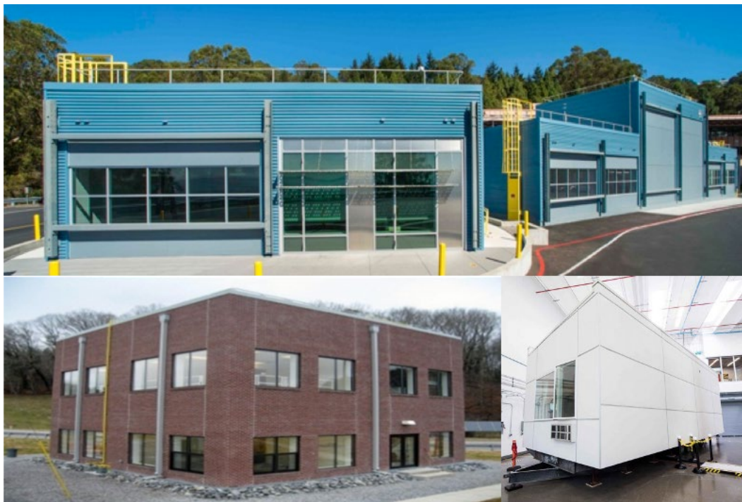
Figure 12. LBNL FLEXLAB (top), ORNL FRP (bottom left), and NREL iUnit (bottom right) test facilities
