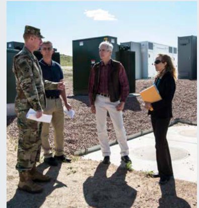
Fort Carson's utility-scale lithium ion battery energy storage system. Photo by Dennis Schroeder, NREL
