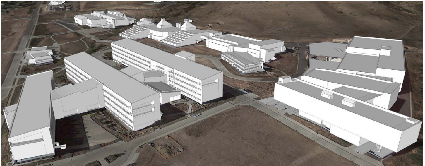
Figure 2. NREL's Intelligent Campus program implemented an EMIS that standardizes data, facilitates reporting, and enables new insights for 33 buildings across two campuses, including its South Table Mountain campus in Golden, Colorado (shown here).
