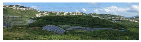
Figure 32. PV system damaged by Hurricane Irma, U.S. Virgin Islands. Note the missing panels in the top left. *Photo by Michael Ingram, NREL*
