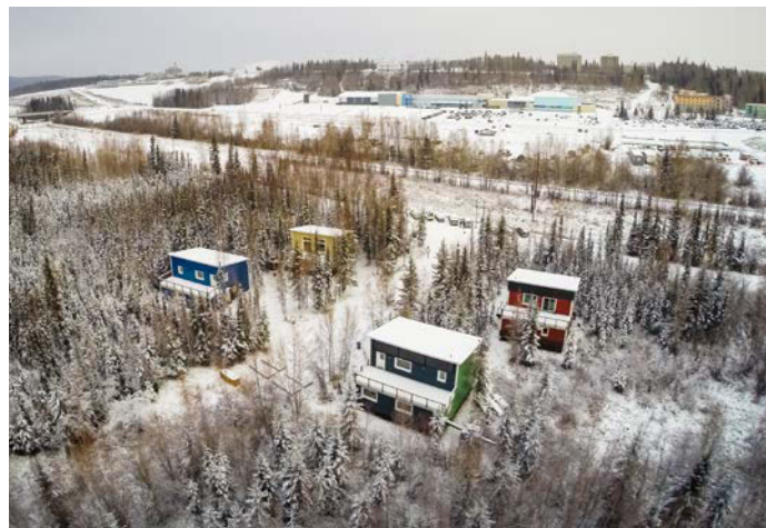
CCHRC built the Sustainable Village at the University of Alaska, Fairbanks in 2012 to create a living laboratory for students and researchers. The four homes each use different combinations of foundations, wall assemblies, and heating and ventilation systems. They have provided a wealth of data on fuel and water efficiency, user behavior, and the effect of building on frozen ground.
