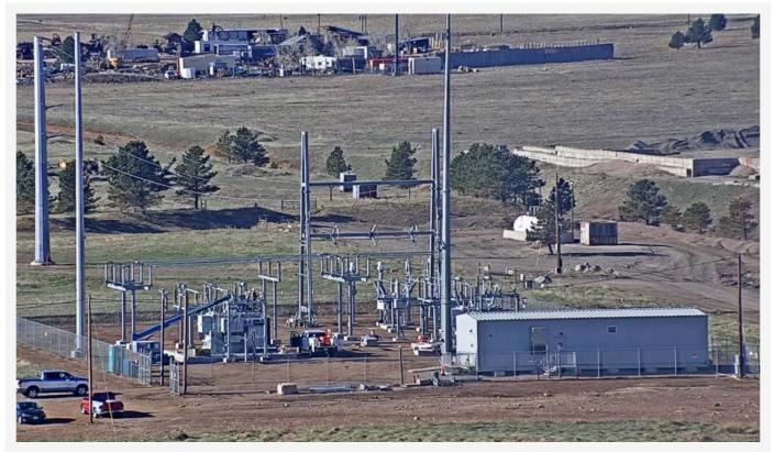
Xcel Energy switchyard civil construction of the 19.9-MW interconnection on the Flatirons Campus. This interconnection further expands research capabilities by allowing researchers to see how grid technologies interact with the larger power grid. *Photo by Brian Cox, NREL*
