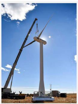
The CART2 with the ARPA-E two-bladed flexible downwind rotor. *Photo by Lee Jay Fingersh, NREL 53511*
