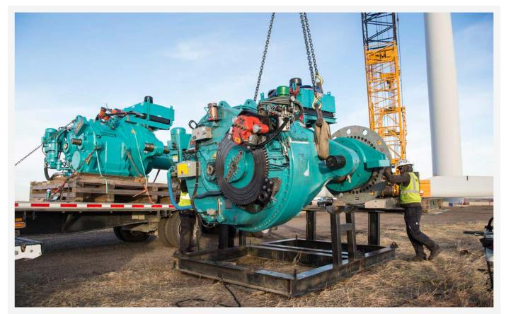
Resolving issues like bearing axial cracking helps to reduce operation and maintenance costs associated with replacing wind turbine parts. Photo by Dennis Schroeder, NREL 49408
