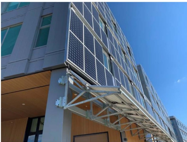
Figure 14. Traditional solar in place of metal cladding on Colorado’s first net-zero multi-tenant building Boulder Commons, Boulder, CO. Photo courtesy of Christopher Klinga.
