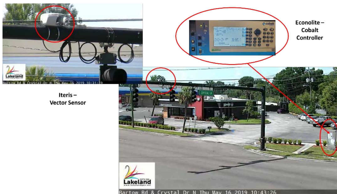
Figure 2. iCASP system with Iteris Vector sensor and Econolite Cobalt controller
