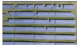
Two images showing various impacts from the same storm in Puerto Rico. Humacao installation (left) suffered near total damage while Oriana array (right) needed replacement of only ~10% of modules, largely because of superior structural design
