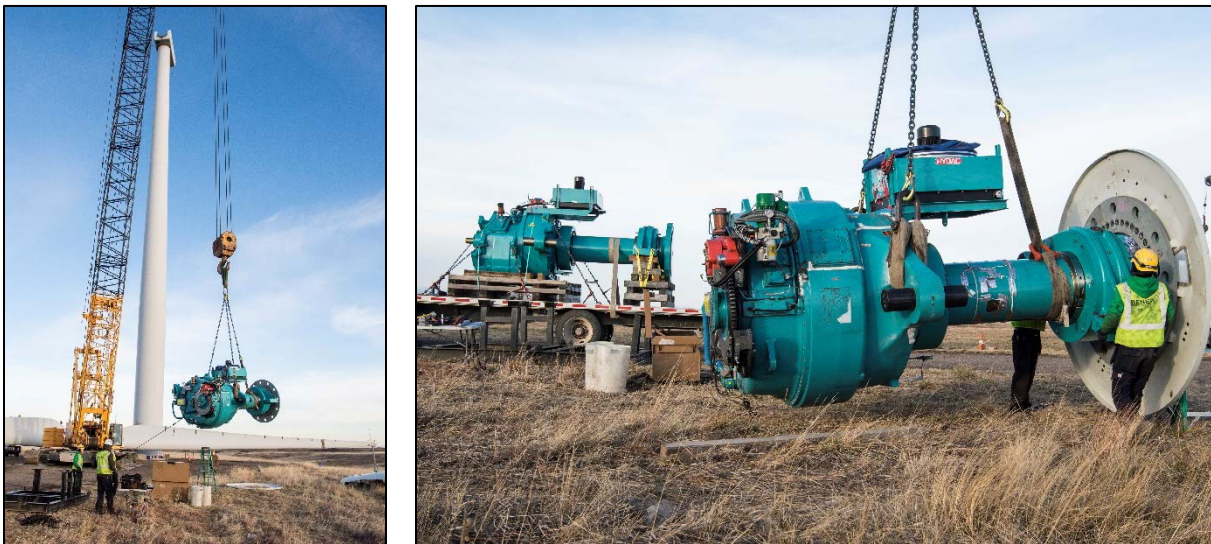
Figure 1. GETS gearbox removal (left) and swap (right) Photos by Dennis Schroeder, NREL 49407 and 49418
