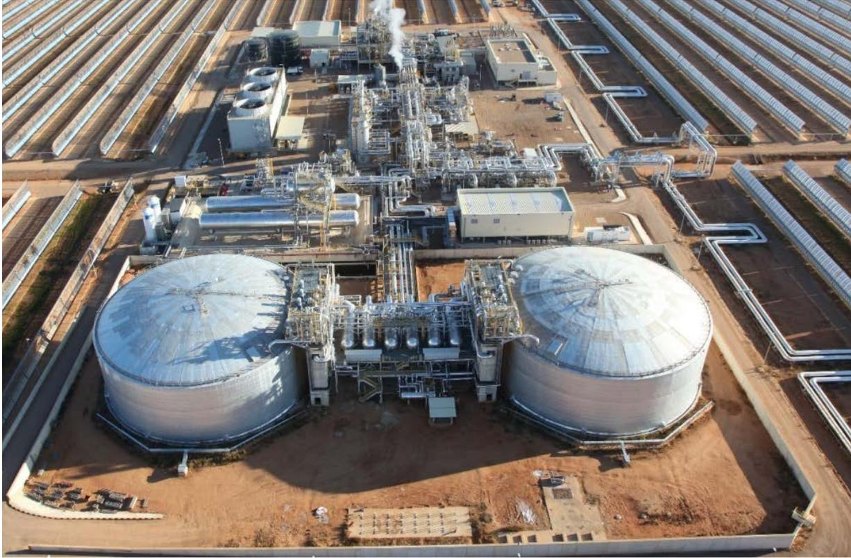
**Figure 5-5. 50-MW Termosol 1 Plant with 9 hours of indirect molten-salt thermal energy storage (Spain)**
