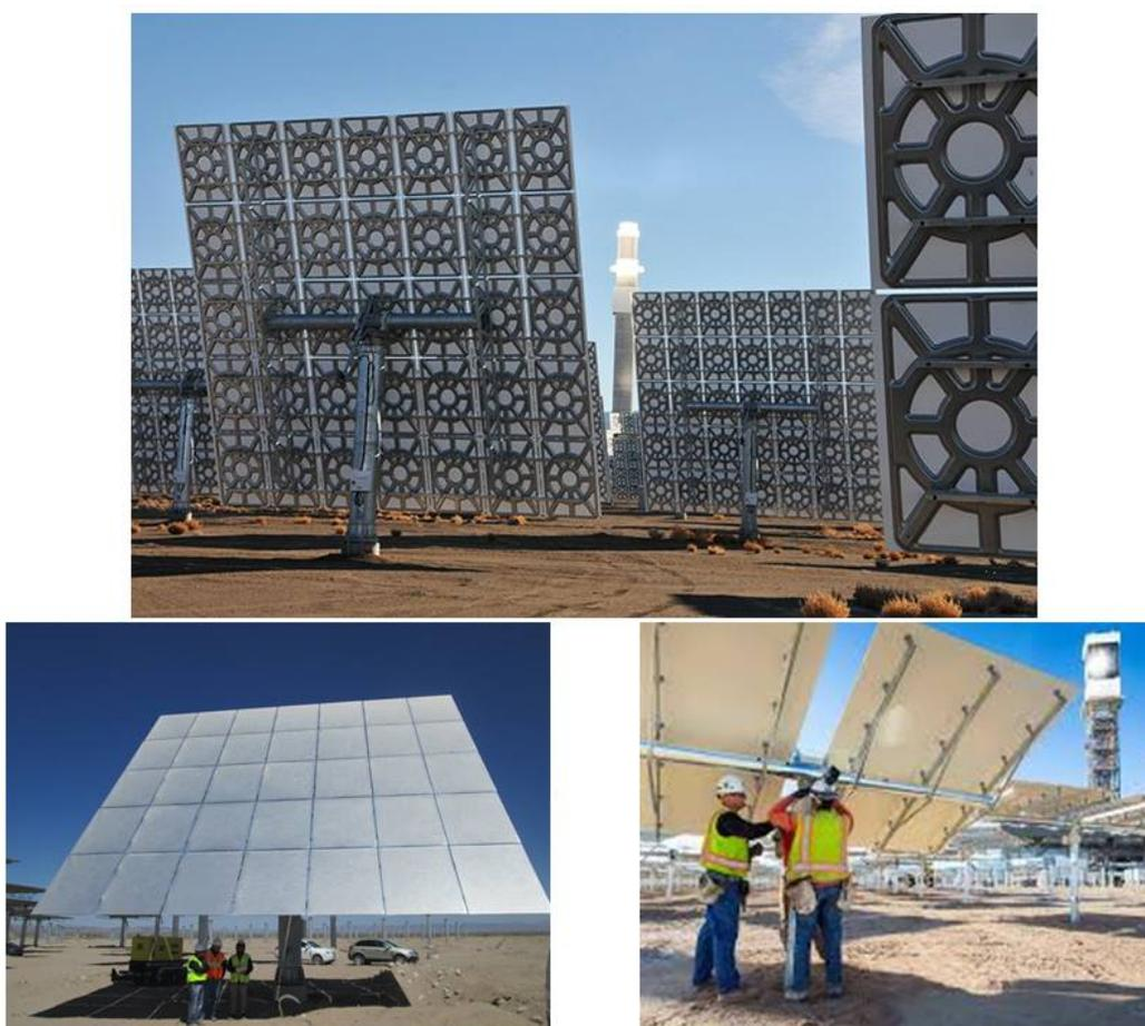
**Figure 6-1. Both large and small heliostats are used in today's commercial power towers**
