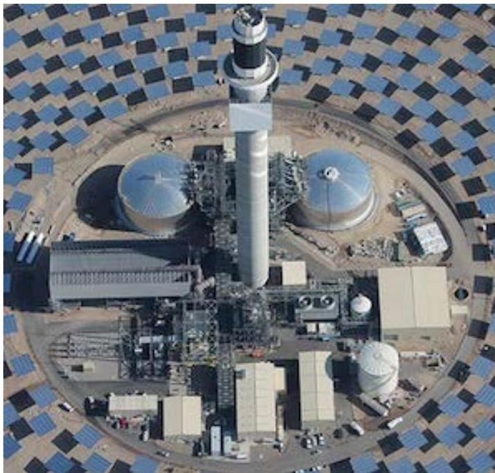
**Figure 6-5. Two-tank thermal storage system at Crescent Dunes**
