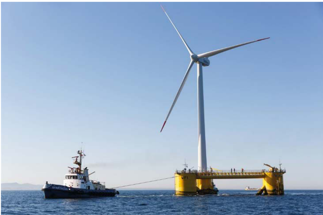
PPI prototype being towed to its station off Portugal in 2011
