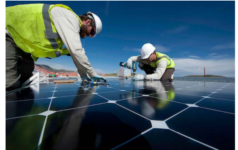
Installation of one of the 3,632 solar modules on NREL's parking garage. The garage can produce up to 1.15 megawatts Photo by Dennis Schroeder / NREL 21487
