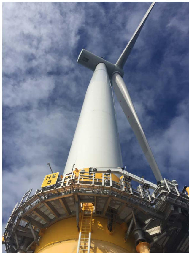
Figure 30. A 6-MW floating wind turbine in Equinor’s 30-MW array near Peterhead, Scotland, supported by a spar buoy floating platform. Photo courtesy of Walt Musial, NREL
