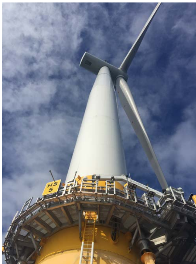
Figure ES-3. A 6-MW floating wind turbine in Equinor’s 30-MW array near Peterhead, Scotland. Photo from Walt Musial, NREL
