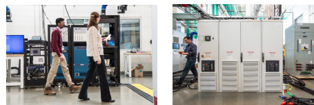
PHIL hardware in NREL's Energy Systems Integration Facility
