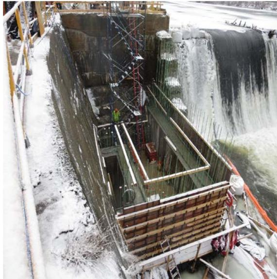
**Figure 3. Glendale Dam Project – Minimum Flow Turbine Replacement. *Photo courtesy of the MassCEC***
