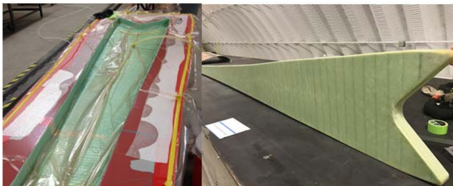
Figure 7. Shear web layup and resin infusion photographs: the infusion process (left), and the finished product (right).
