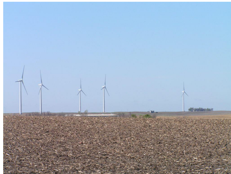
Five GE 1.6-megawatt (MW) turbines at the Junction Hill Top Wind Farm in Iowa. Photo by Tom Wind, NREL 26494
