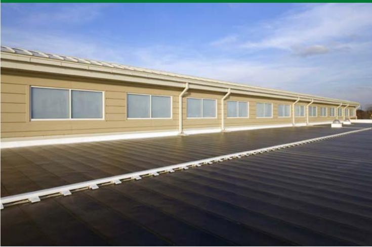
The energy efficiency measures incorporated into Richardsville Elementary School in Bowling Green, Kentucky, reduced its annual EUI to 18.2 kBtu/ft<sup>2</sup>·yr, making it possible to get to zero energy with this rooftop photovoltaic system (see the “Achieving Net Zero: Richardsville Elementary School” case study in Helpful Resources). *Photo by Rachel Paul Photography, NREL 18603*
