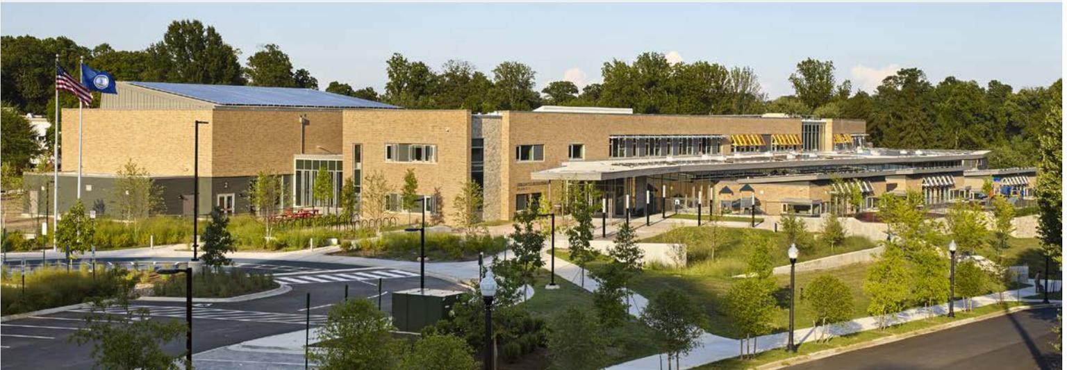
Designers of Discovery Elementary School in Arlington, Virginia, oriented the building on an east-west axis to optimize solar exposure for the future PV system and maximize daylighting without creating glare (see the *Discovery Elementary: Zero Energy Is an A+ for Education* case study in Helpful Resources). *Photo from VMDO Architects/©Alan Karchmer*
