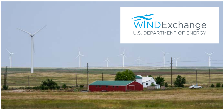
Cedar Creek Wind Farm in Grover, Colorado. Photo by Dennis Schroeder, NREL 30585
