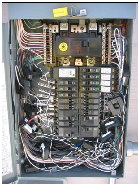
Figure ES1. Conventional submetering installed inside a residential electrical panel.
