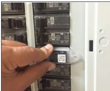
Figure 8. Stencil used to ensure proper placement of the sensor on the breaker
