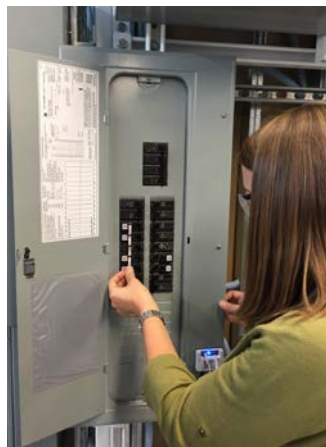
Figure 10. Step 2 – Use ribbon cable to connect all sensors to the hub
